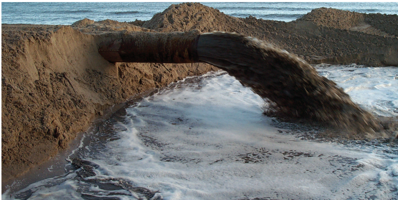
Sediment is pumped into areas for shoreline stabilization. Image: CWPPRA
