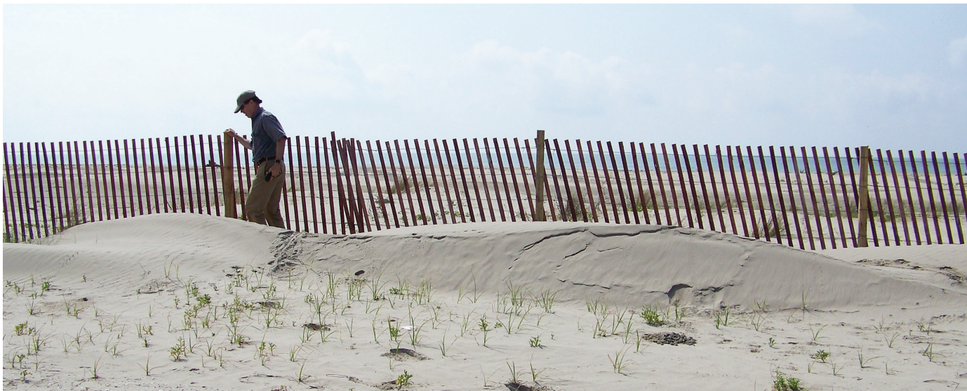
Sand fencing captures wind-blown sediment. Image: CWPPRA
