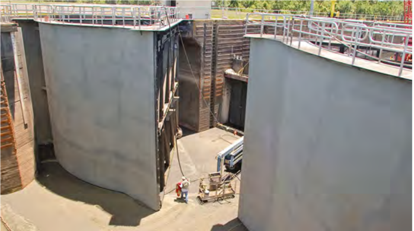
Work on the Algiers Lock in New Orleans. Workers descend on the dewatered structure to complete repairs. U.S. Army Corps of Engineers. Image: Kirk Dietrich.
