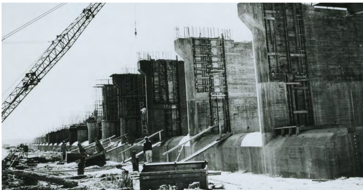
Construction of the Morganza Spillway. Image: U.S. Army Corps of Engineers.
