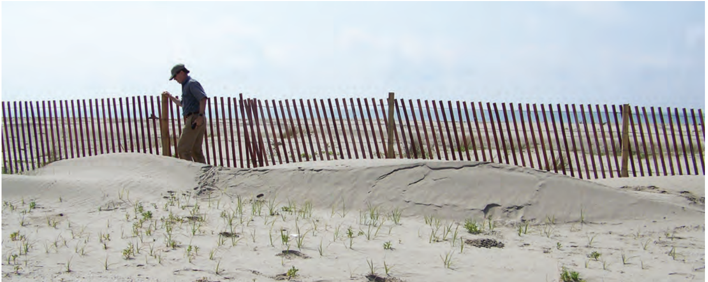
Sand fencing captures wind-blown sediment. Image: CWPPRA
