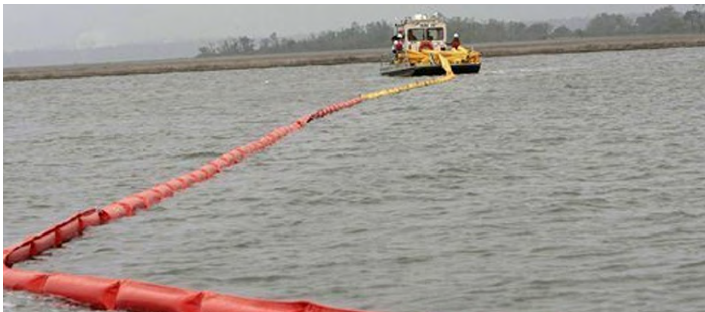
Boom is deployed to protect fragile marshland during an oil spill. Image: NOAA
