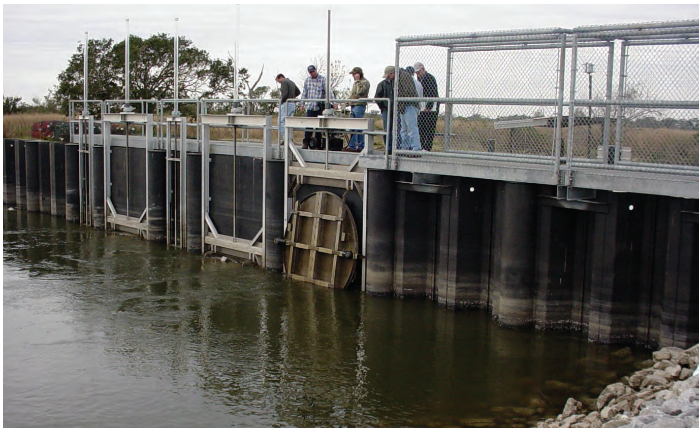
Circular flap gates control water flow. Image: CWPPRA
